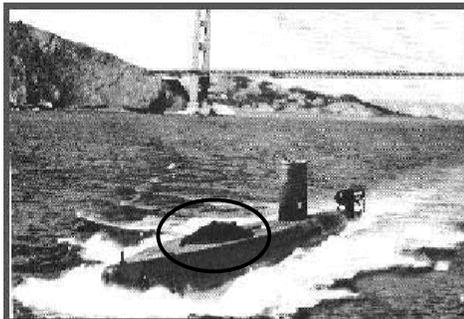
USS Halibut with disguised chamber for diving
